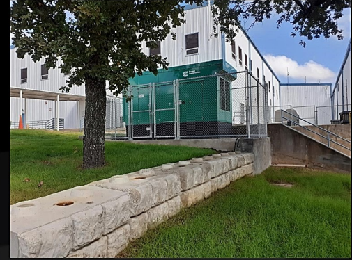
FEMA – Emergency Generator Installation Denton, Texas
